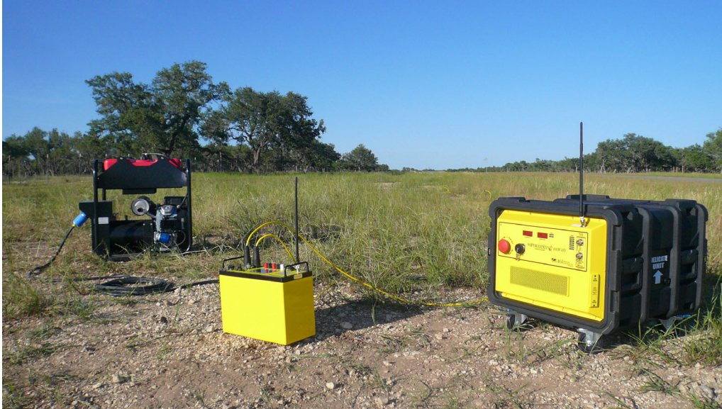
Figure 37: The SGS generator, SuperSting R8, and a PowerSting make up the system.
